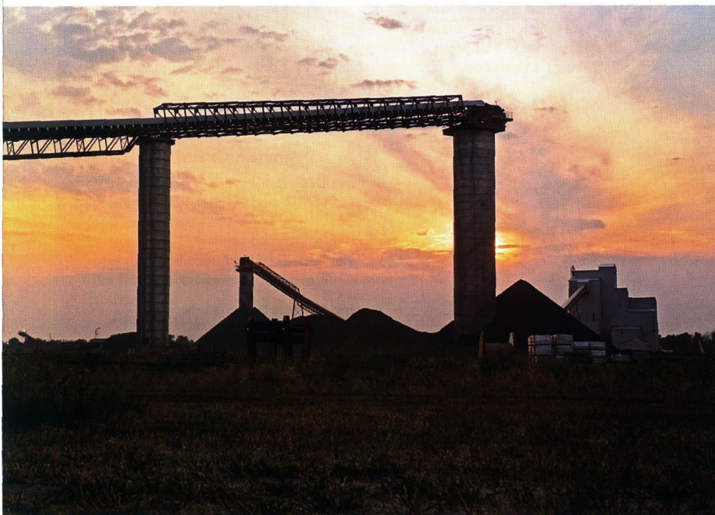
Surface coal handling conveyors
